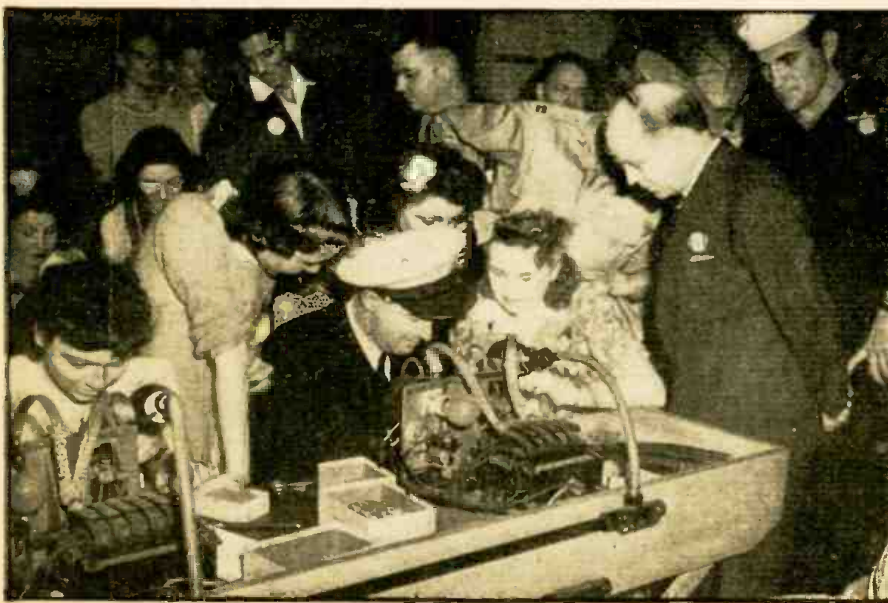
Chief Metalsmith Ed Regan (U. S. Navy) receives detailed instructions on a new and secret tube-welding process from an employee of National Union Radio Corporation.
